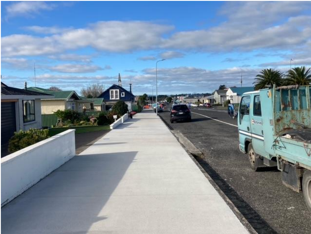
Figure 3 – Footpath replacement on Regan Street.
