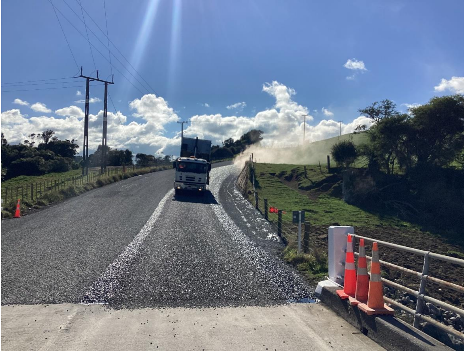
Figure 5 – Sealing of Palmer Road following the re-build of the road pavement.
