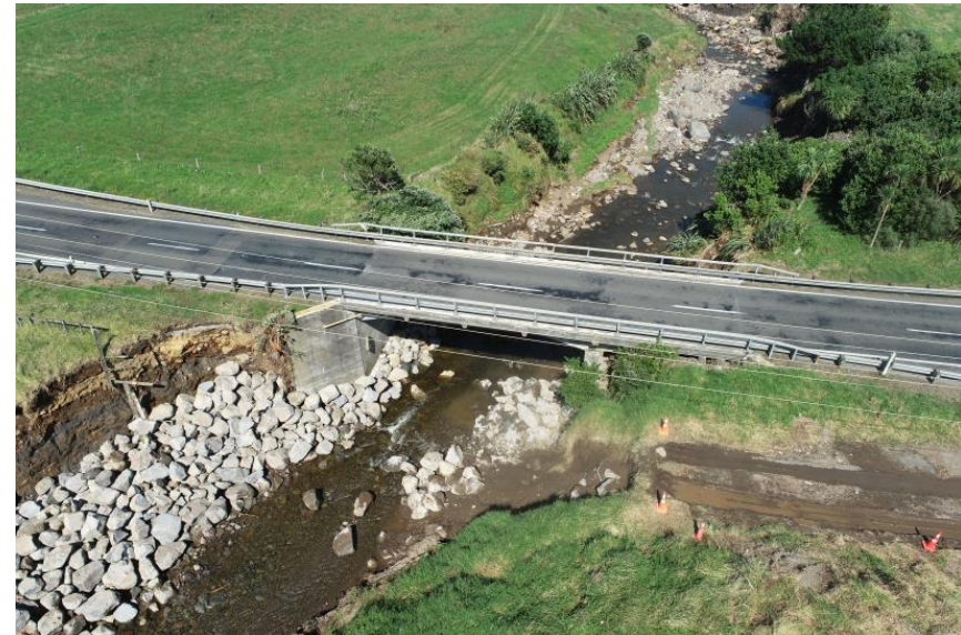
Heimama Stream Bridge
