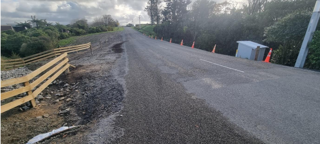
Figure 7 – Monmouth Road reinstated and resealed to be opened on 4 April.
