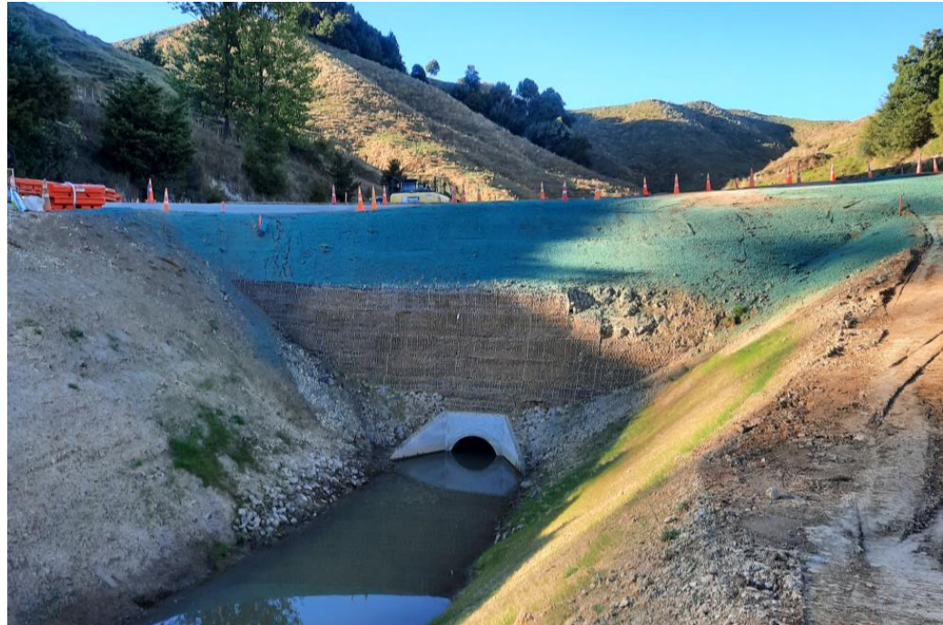
Tahora Saddle Culvert
