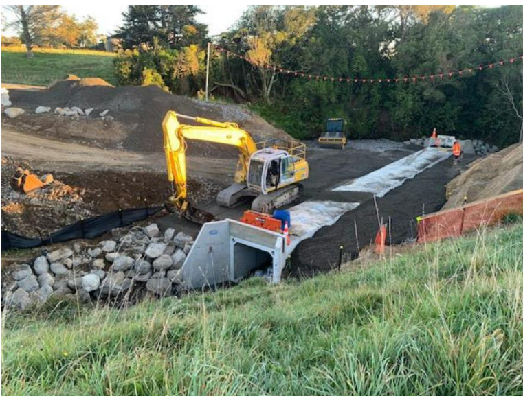
Figure 6 – The new culverts have been installed with backfilling being done.
