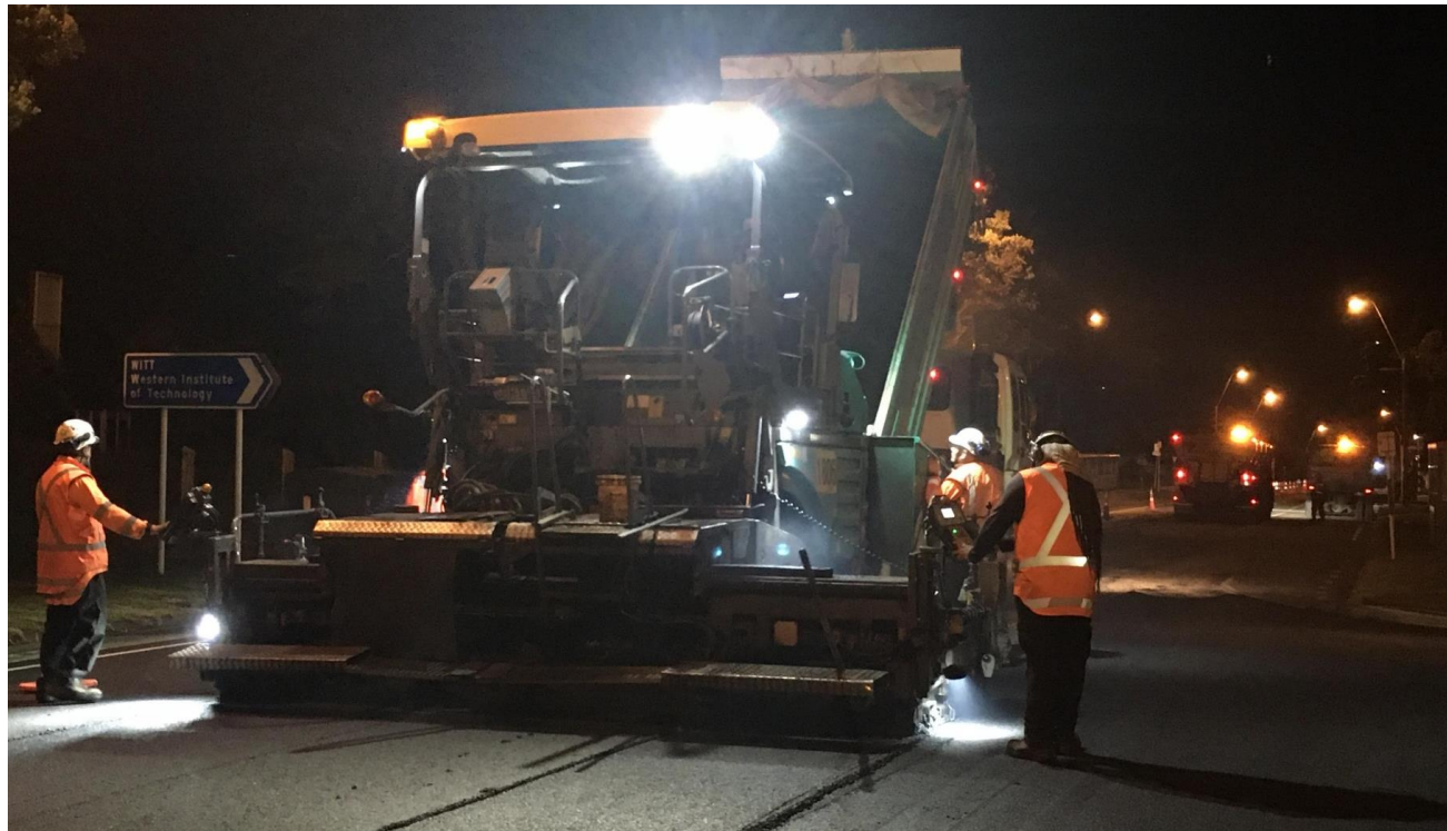
Asphalting SH3 (Coronation Ave) in New Plymouth
