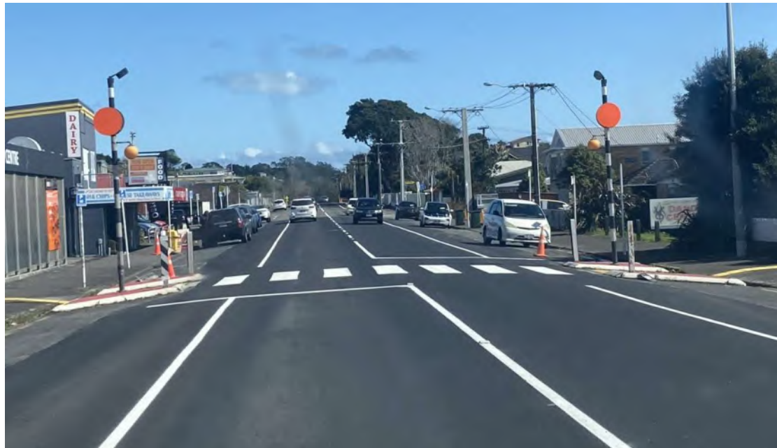
Completed asphalt site SH44 New Plymouth
