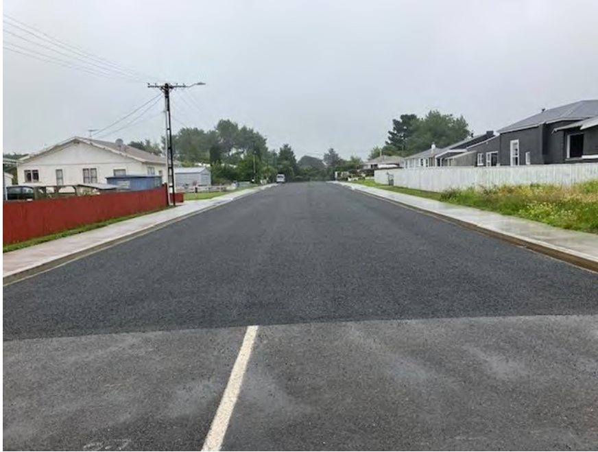
Figure 1 – Footpath replacement on Elsinore Street.
