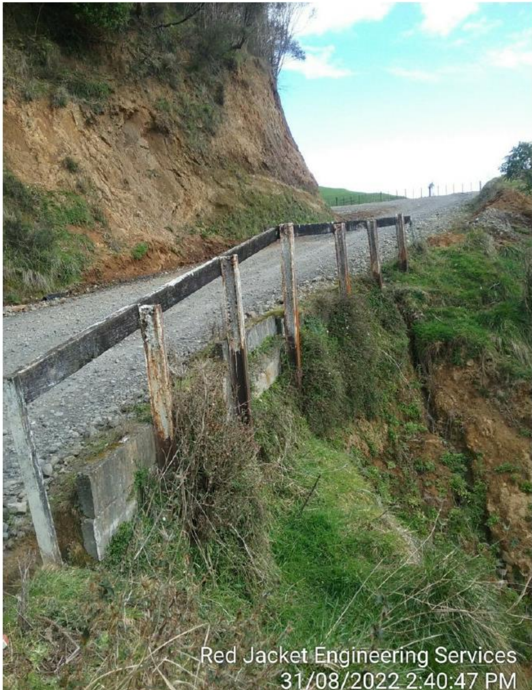
Figure 3 – Douglas North Rd retaining wall.
