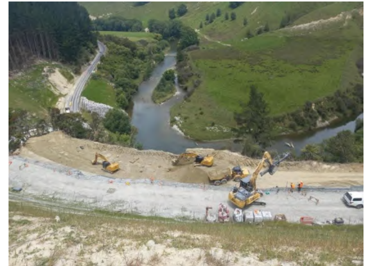
Auraki Stream Road Retreat site – looking south from the top benches.
