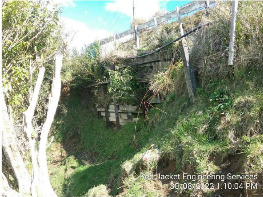
Figure 2 – Croydon Rd retaining wall.
