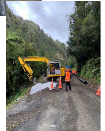
Culvert replacement and shoulder works underway
