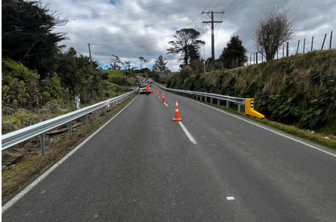
Figure 2 – The new barrier installed at Mangatoki Stream on Opunake Road.
