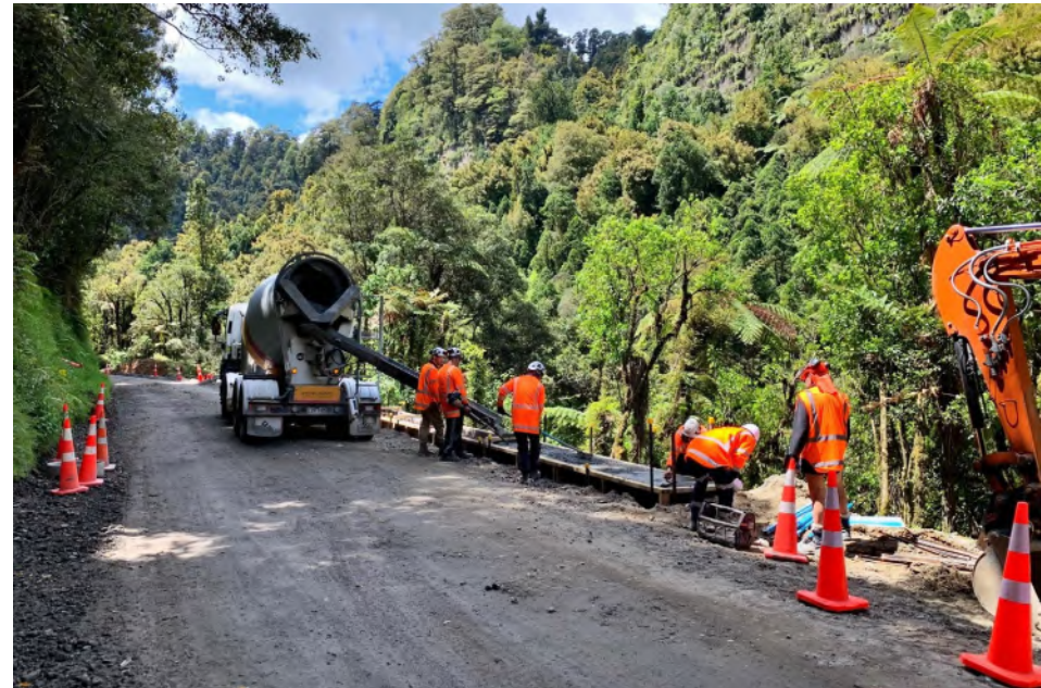
Work underway in the Tangarākau Gorge
