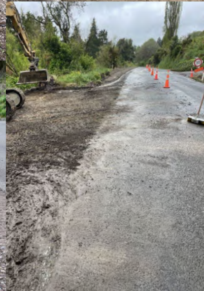
Bridge dropout repair
