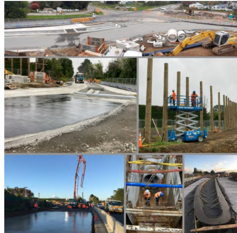
Work underway at Princess Street intersection
