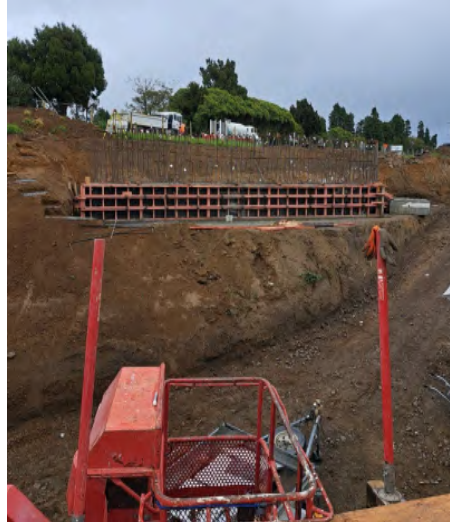
Abutment - concrete pour completed
