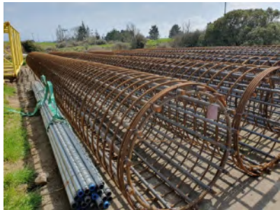
Reinforcing cages for piles and columns
