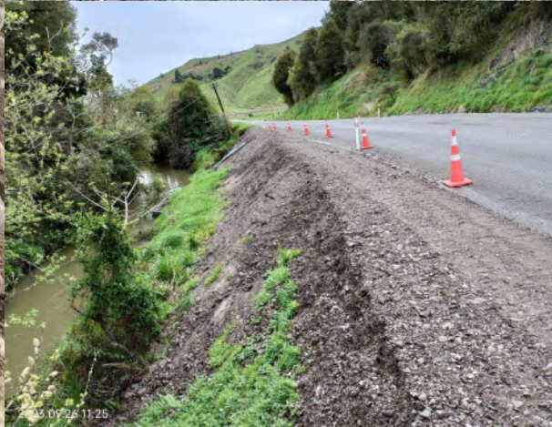
Tatu dropout repair
