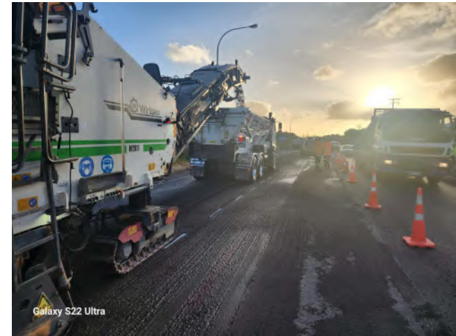
Work underway at Bell Block Mangaiti Road
