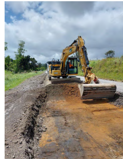
Work underway on SH3A Osflo
