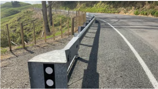
Newly installed barrier near Roto Rd in Aukopae
