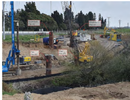
View of site from abutment
