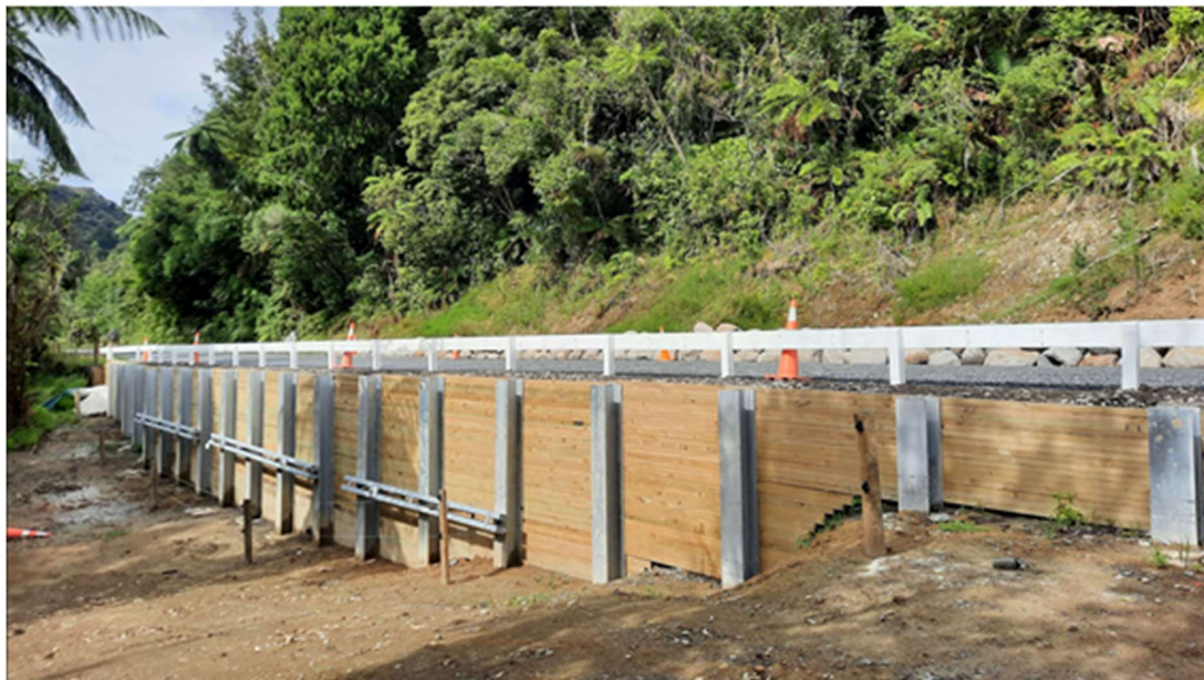
Picture - Okau Road retaining wall
