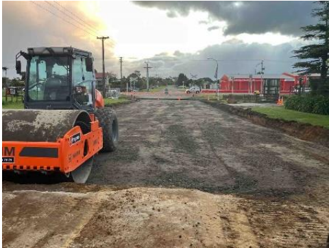
Figure 3: Flint Road East – Basecourse placed and compacted to form the road foundation.
