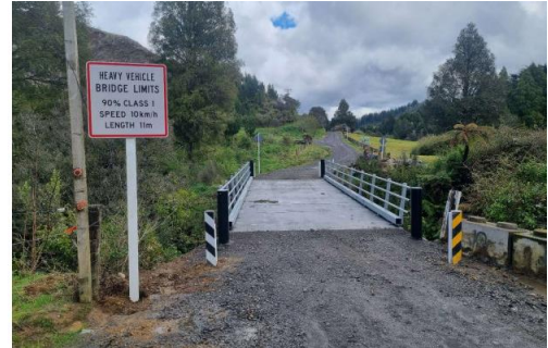
Figure 7: The completed bridge.
