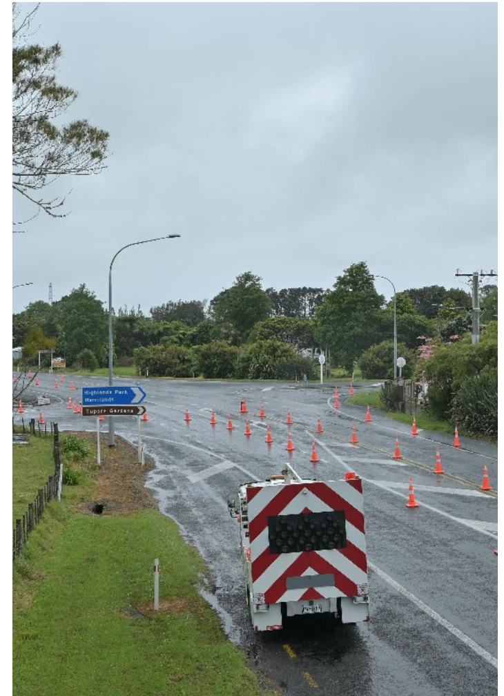
Image: Works underway at Mangorei Road intersection
