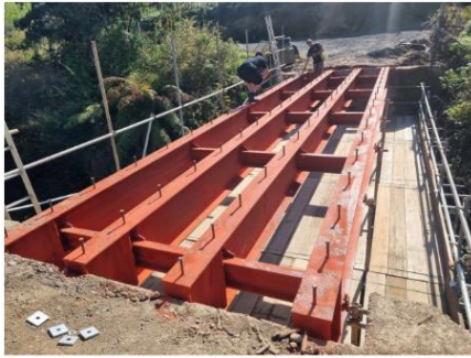
Figure 6: New steel beams installed to support the concrete bridge deck.
