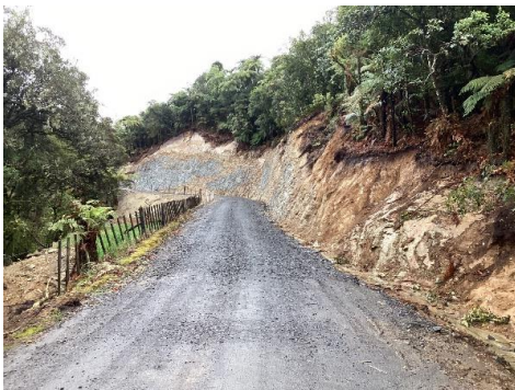
Figure 8: Bank retreat on Junction Rd.
