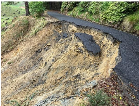
Figure 10: Mohakau Rd - Before and after.
