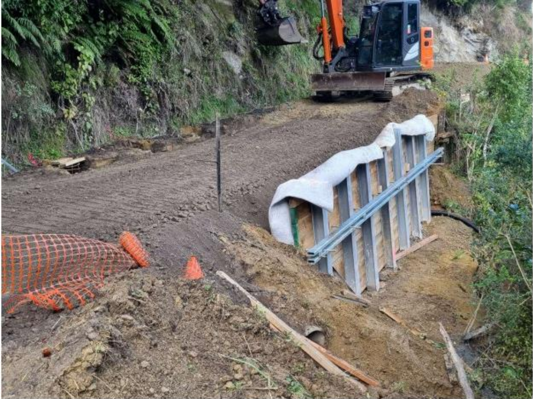
Figure 6: Repairs to the wall on Junction Rd located at RP12.60.
