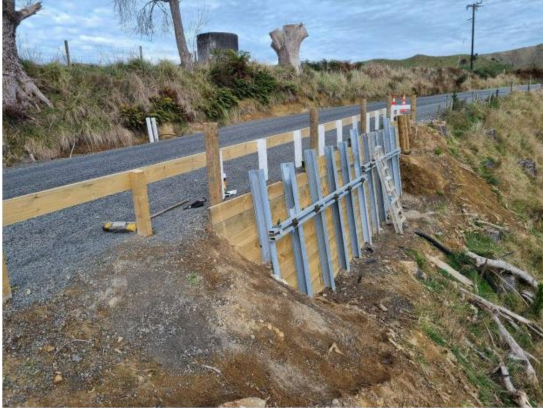
Figure 8: Replacement wall on Mangaotuku Rd at RP5.00
