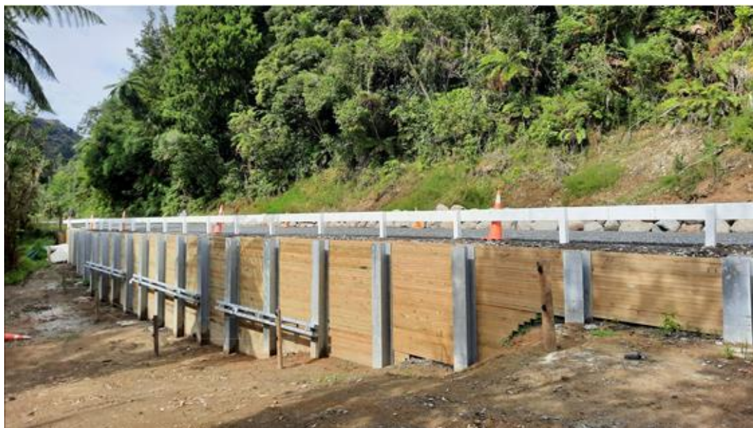
Picture - Okau Road retaining wall
