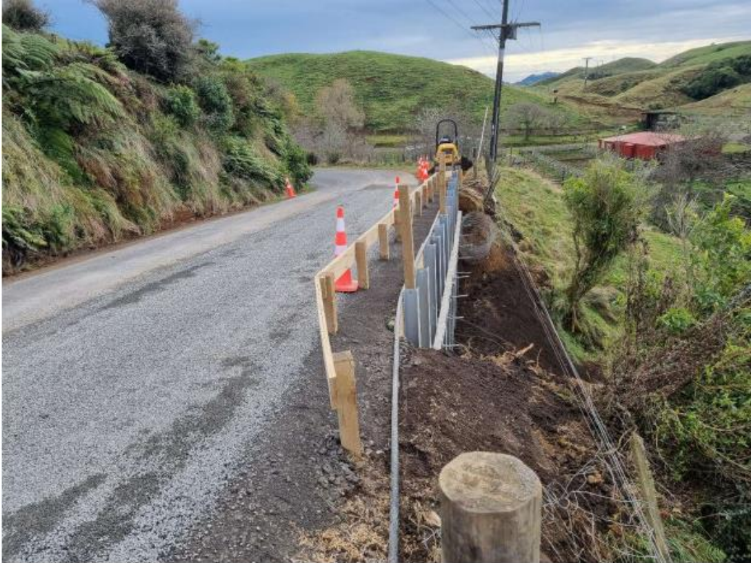
Figure 7: Replacement retaining wall on Croydon Rd at RP11.86
