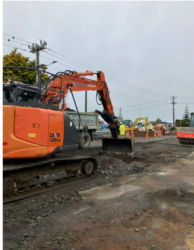
Pavement and sub soil drainage works.
