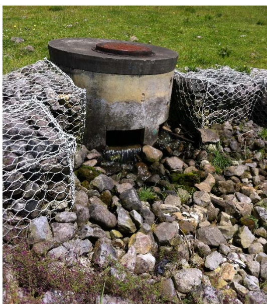
FIGURE 6: Rock Filter Outfall
