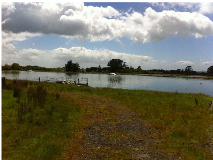
FIGURE 4: Oxidation Pond – Pond 1
