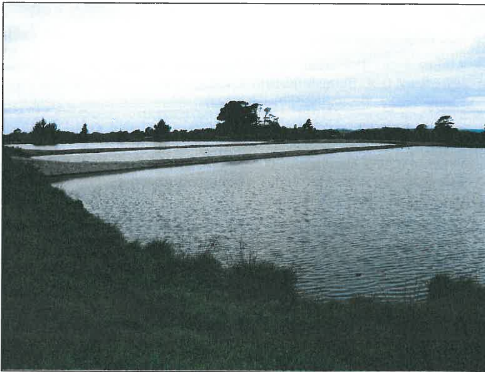
Figure 1: Photo illustrating the three cells of oxidation Pond 2
