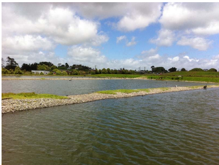
FIGURE 5: Maturation Pond – Pond 2
