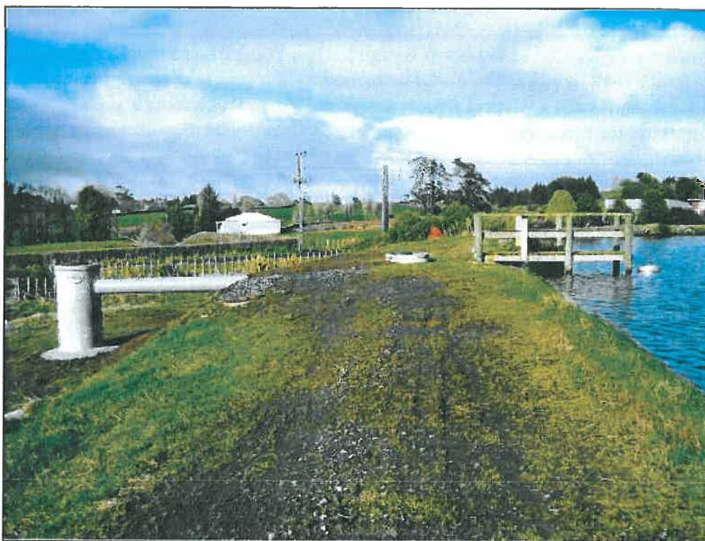
Figure 2: Photo illustrating the re-engineered outlet structure
