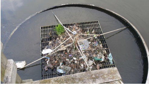
Photo 1 & 2 Primary pond outlet, December 2014 and June 2015
