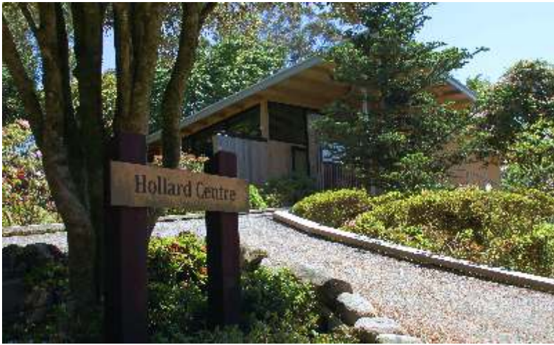
'A pavilion of natural materials which nestles into the surrounding natural environment ...'
