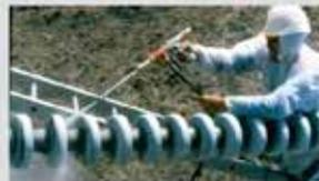
Ash is cleaned from a 110 kV horizontal insulator string using pressurised water following the 1905 Ruapehu eruption, New Zealand (Transpower New Zealand)
