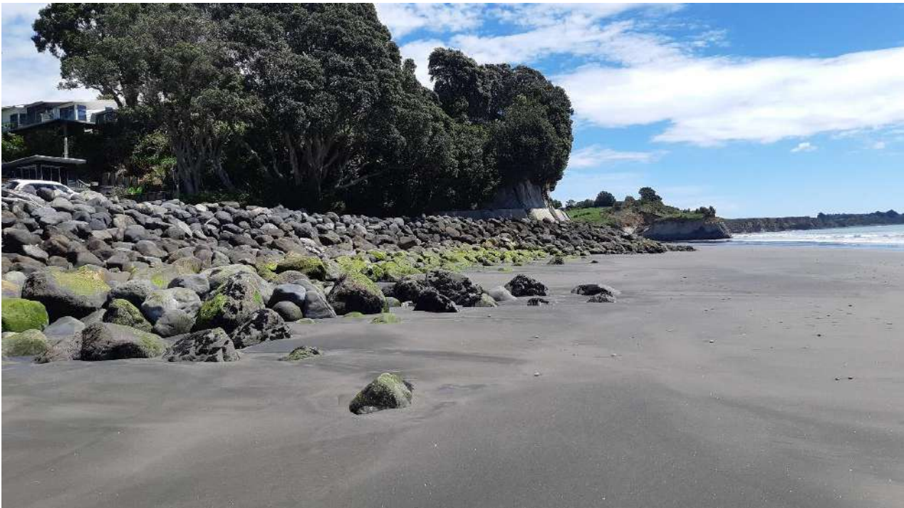
Figure 13 Photograph showing rock revetment along New Plymouth coastal walkway with backdrop of vegetation.
