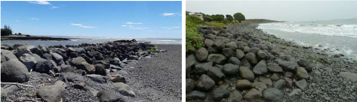
Figure 12 Photographs showing examples of colour, form and character of local rock revetment in context of beach and river environments.
