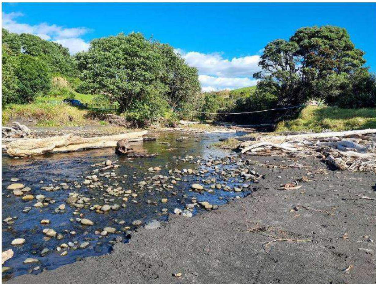
Figure 20 Photograph showing the previous swing bridge in place (with the white line being the water pipe running under the platform of the bridge).
